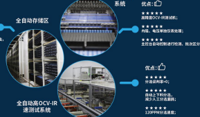
存储/OCV/分选系统 Automatic OCV And Sorting System
